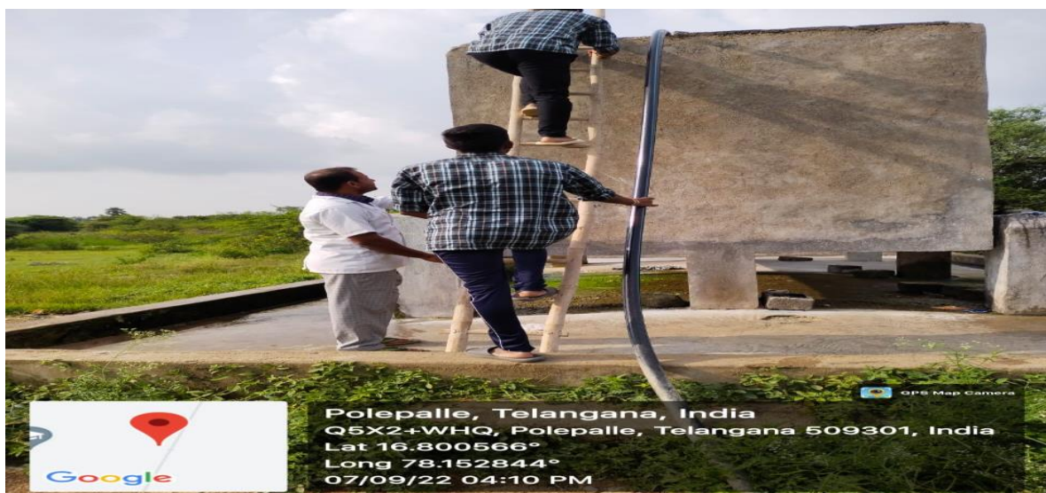
Cleaning of overhead Tank
