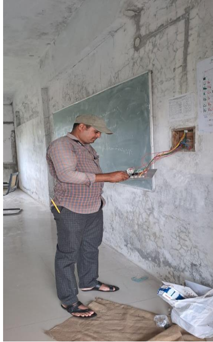
Electrician checking for loose connections
